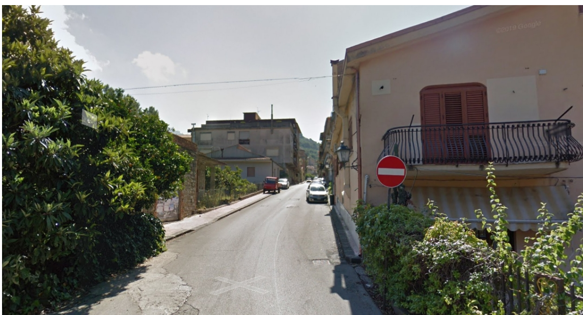
SP. 146/a dik Ponte Naso – Sinagra Km 11+900
