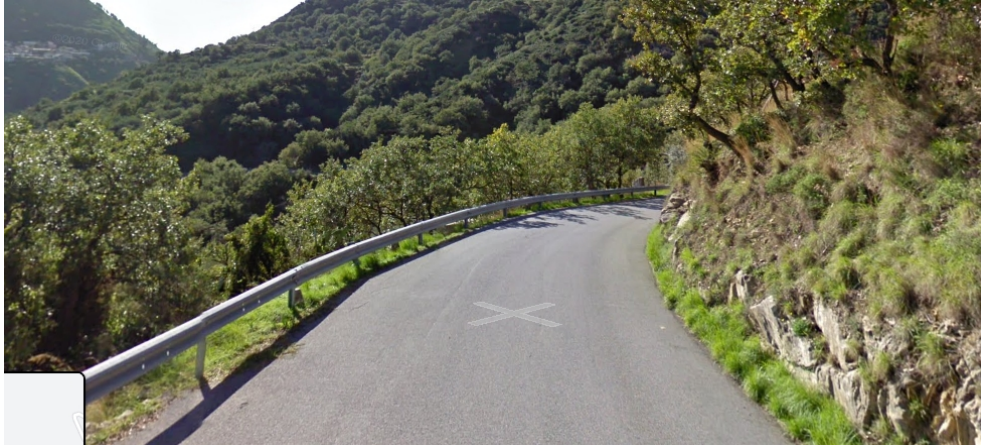
SP.115 INTERVENTO 3 Km 2+790
